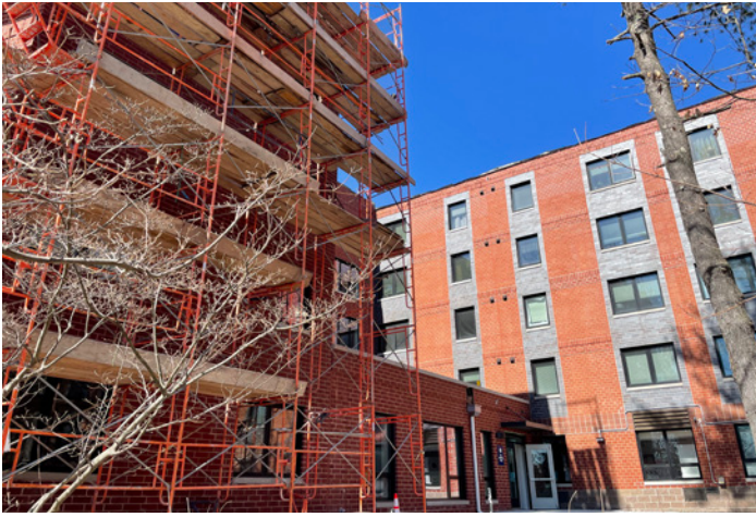
Coleman House Retrofit
